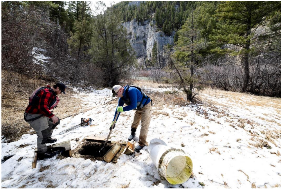
Volunteers dismantling and filling old latrine hole.
