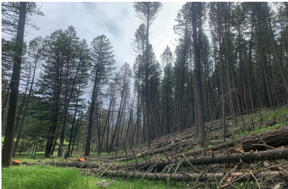
Hazard Tree Mitigation At Lower Trout Creek Boat Camp
