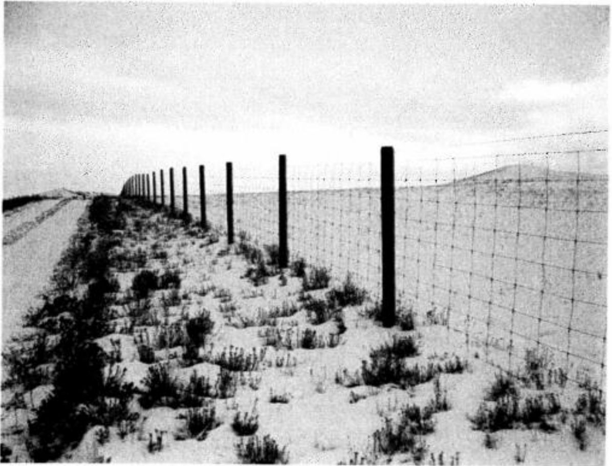
Figure 2. Bison quarantine fence. Note the high tensile page wire and top high tensile wire. Fence height is 8' with wooden brace posts every 15feet.
