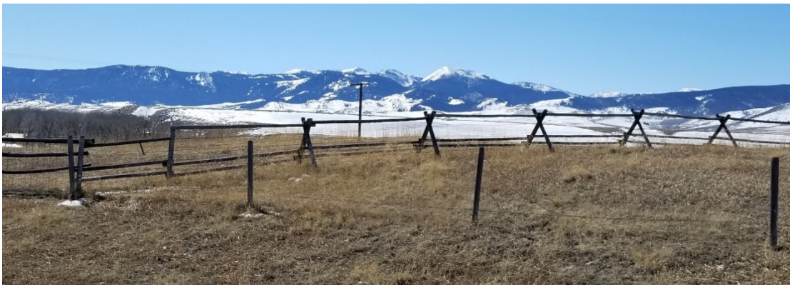
Figure 2.9. The problematic fencing barrier between Highway 287 and the Madison River. The jack-leg fence and wire combination resulted in a fence impassible to pronghorn. Photo credit: BLM
