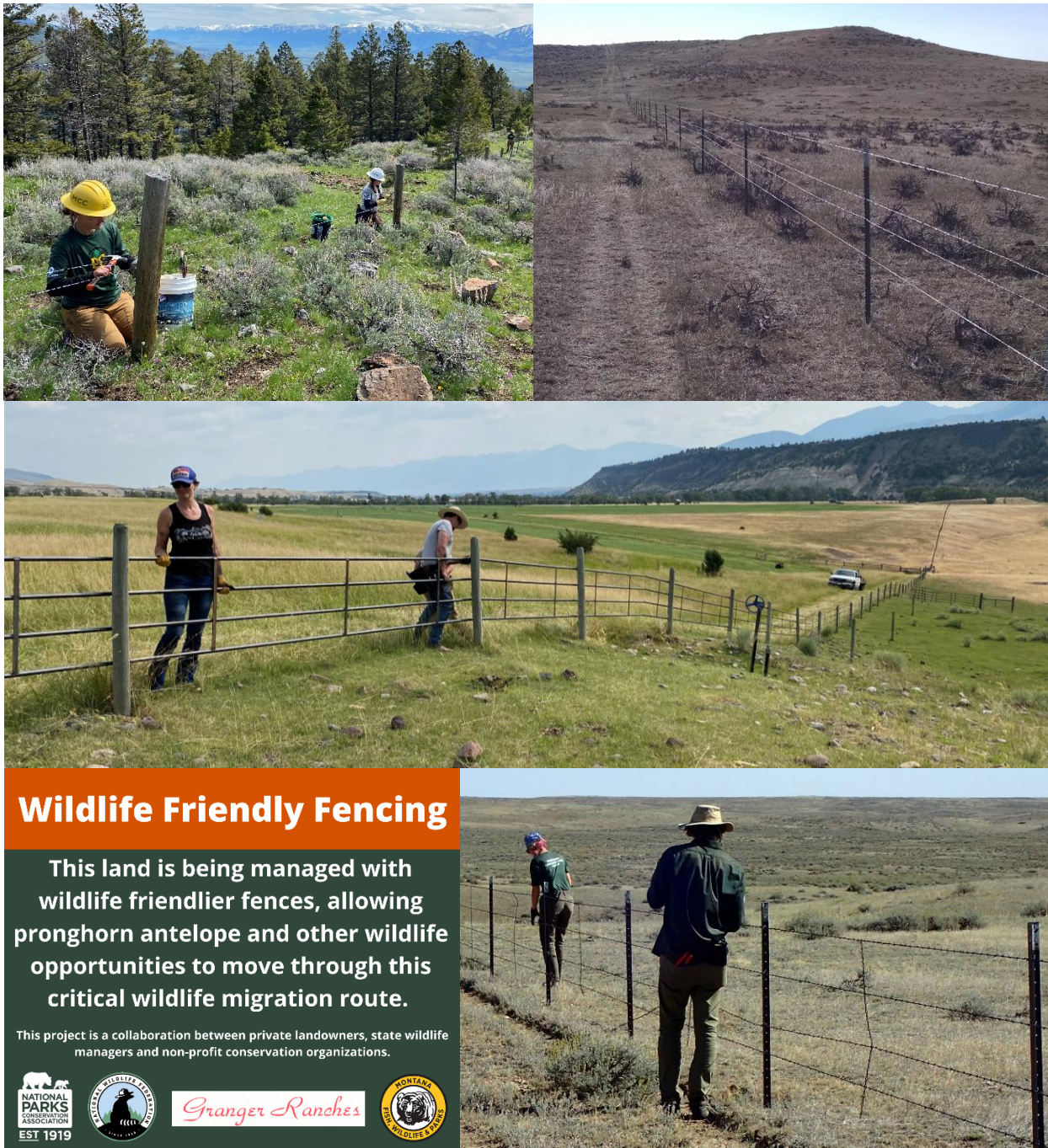
Figure 67. Examples of fence modification projects informed by the pronghorn collar data and completed by partners of the Montana Pronghorn Movement and Population Ecology Project. Top left photo: modifying a 5-strand fence to a 4-strand fence with smooth bottom wire in the Paradise study area (photo credit: National Parks Conservation Association). Top right photo: new 4-strand fence with smooth bottom wire replacing 5-strand barbed wire fencing in the Fergus-Petroleum study area (photo credit: BLM). Middle photo: installing metal panels to replace 5-strand barbed wire fence in the Paradise study area (photo credit: National Parks Conservation Association). Bottom left image: signage used for outreach in the Madison study area. Bottom right photo: removing barbed bottom wires in the South Philips study area (photo credit: BLM).
