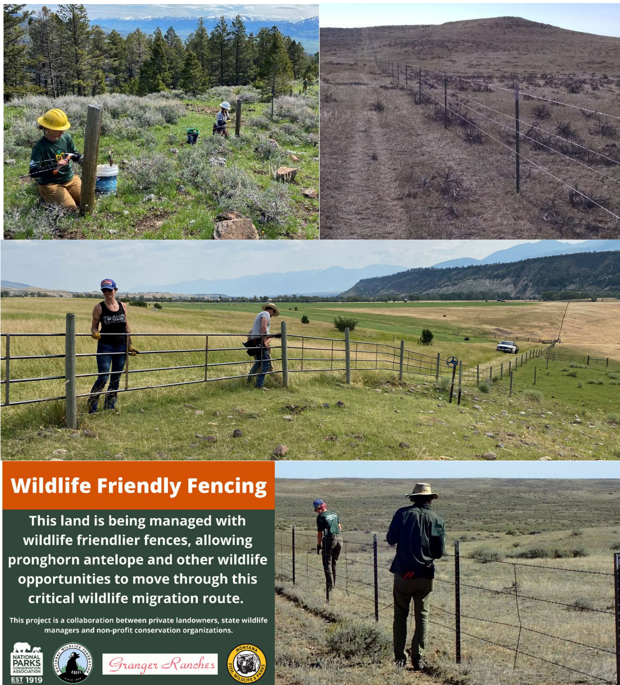
Figure 51. Examples of fence modification projects informed by the pronghorn collar data and completed by partners of the Montana Pronghorn Movement and Population Ecology Project. Top left photo: modifying a 5-strand fence to a 4-strand fence with smooth bottom wire in the Paradise study area (photo credit: National Parks Conservation Association). Top right photo: new 4-strand fence with smooth bottom wire replacing 5-strand barbed wire fencing in the Fergus-Petroleum study area (photo credit: BLM). Middle photo: installing metal panels to replace 5-strand barbed wire fence in the Paradise study area (photo credit: National Parks Conservation Association). Bottom left image: signage used for outreach in the Madison study area. Bottom right photo: removing barbed bottom wires in the South Philips study area (photo credit: BLM).
