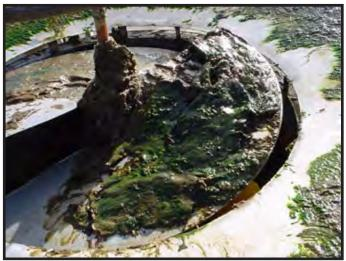
SolarBee With Buildup On Impeller
