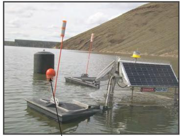
Anchor Chain Connection Point (At Float Ball)
