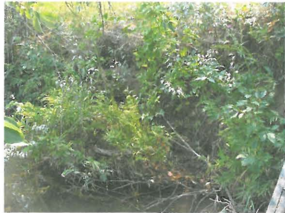
Same view taken this July. This is caused by boat wakes. (July 2021)
