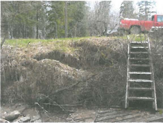
Slough bank near our boat house(for row boat), a large chunk of bank has broken off. (Spring 2020)
