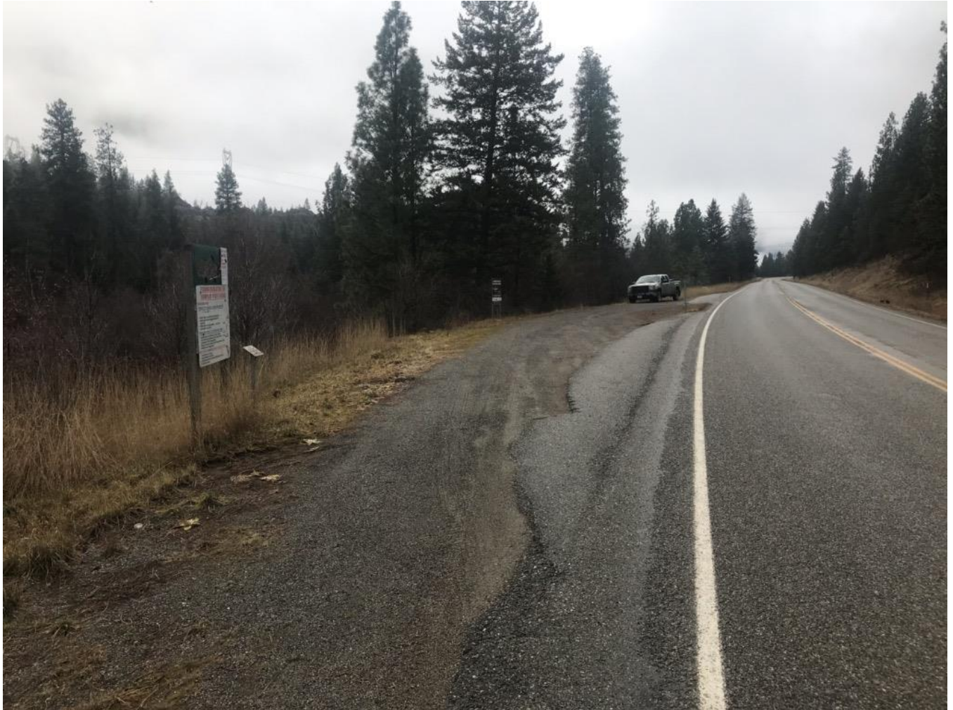
Figure 5. The existing parking area on a county road right-of-way just upstream of the proposed FAS and adjacent to United States Forest Service land. Two FWP signs already exist at this parking area.
