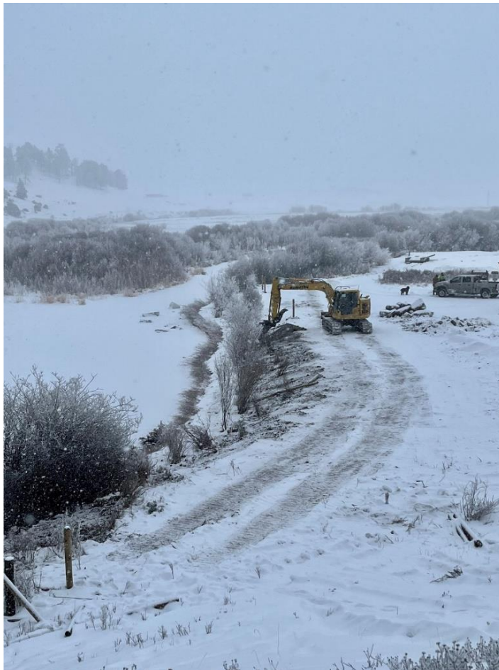
Bioengineered Bank Restoration at Former Downstream Boat Ramp
