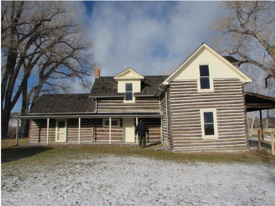
Figure 15: South elevation of the Chief's House at Chief Plenty Coups State Park. The uneven settling caused by foundation issues is clearly visible in the crooked gable end.
