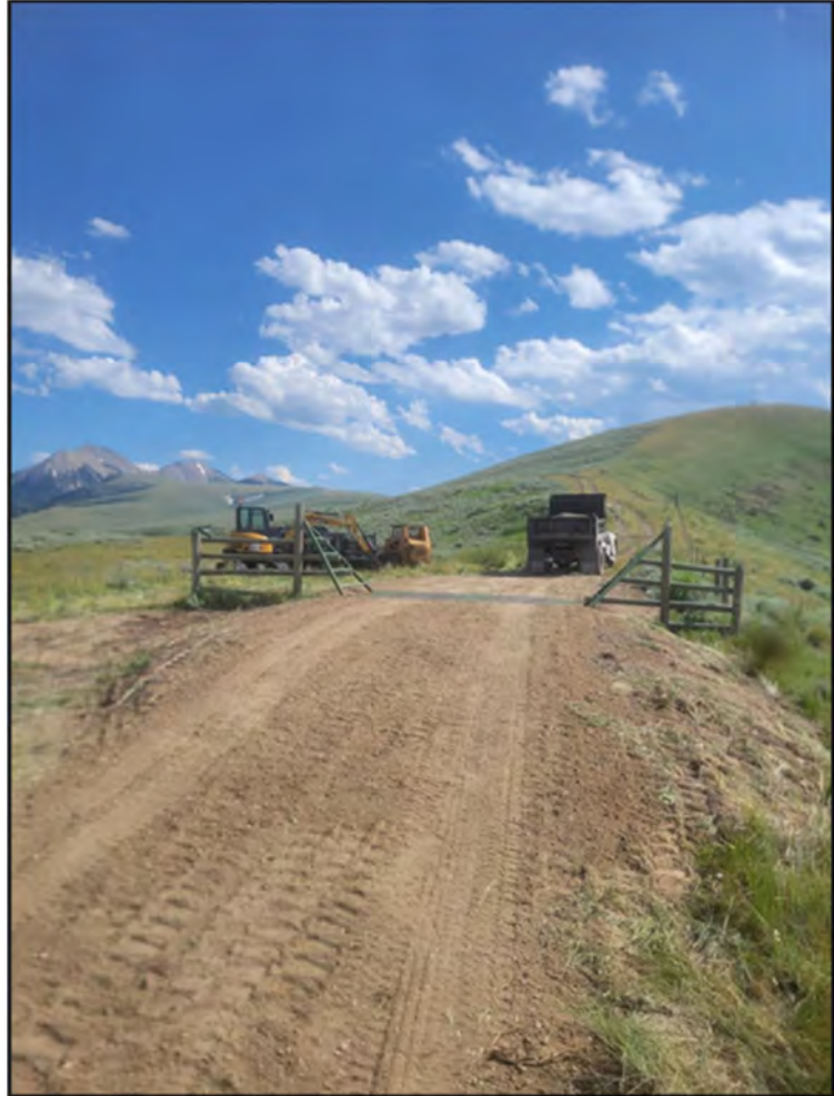
New cattle guard installation, Blacktail Wildlife Management Area, 2023. (Image: Paul Peterson).
