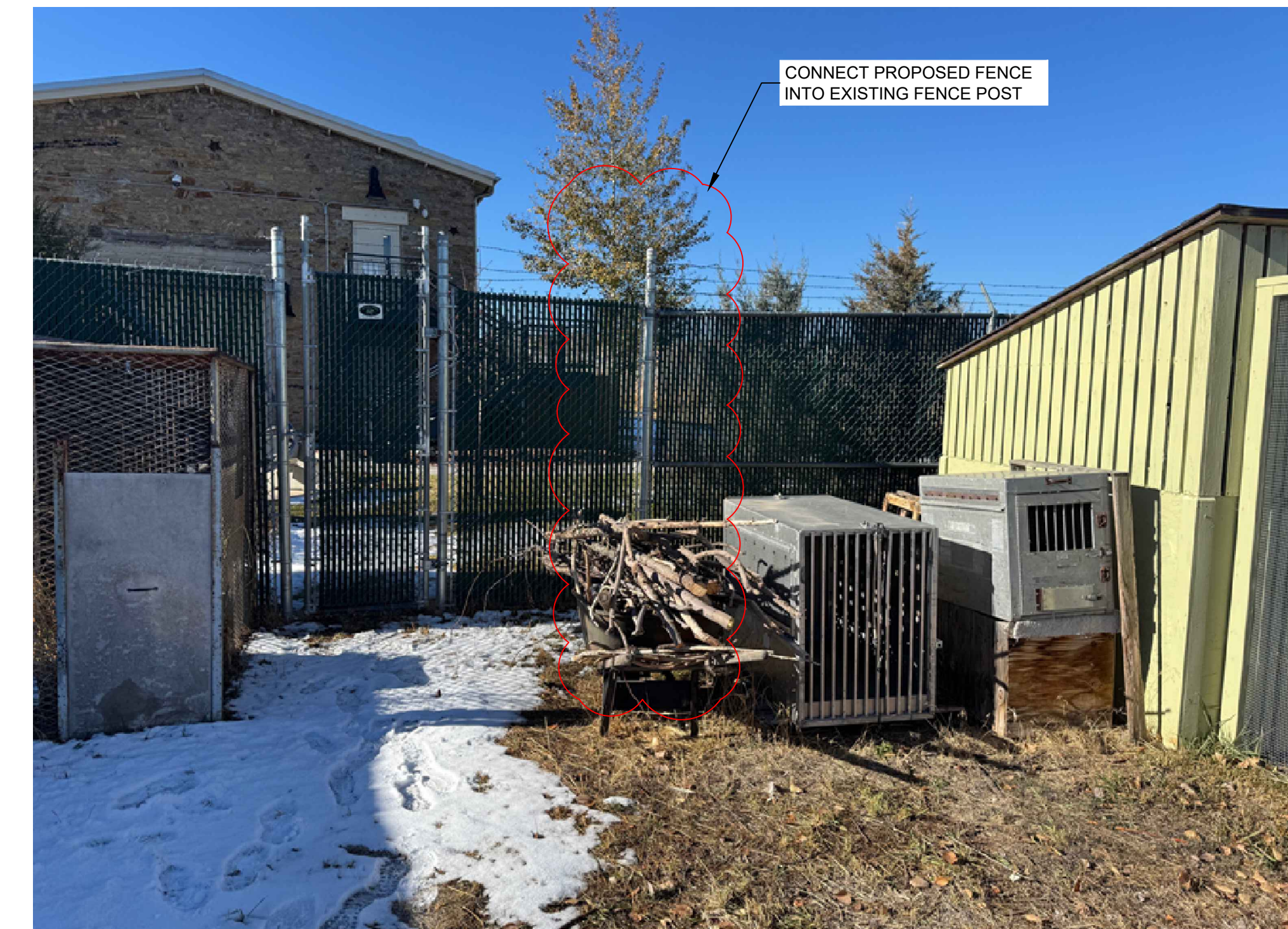
1 CS002 NTS FENCE POST CONNECTION LOCATION
