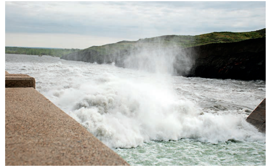
THAR SHE BLOWS! Massive snowmelt and heavy rains in spring 2011 forced the U.S. Army Corps of Engineers to release a record 90,000 cubic feet of water per second through the Fort Peck spillway in mid-June. Shown here: 50,000 cfs on June 11.
