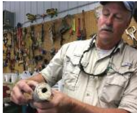
CLOGGED Lewis & Clark Caverns maintenance supervisor Bill Foreman shows a restroom septic pipe filled with mineral scale.
