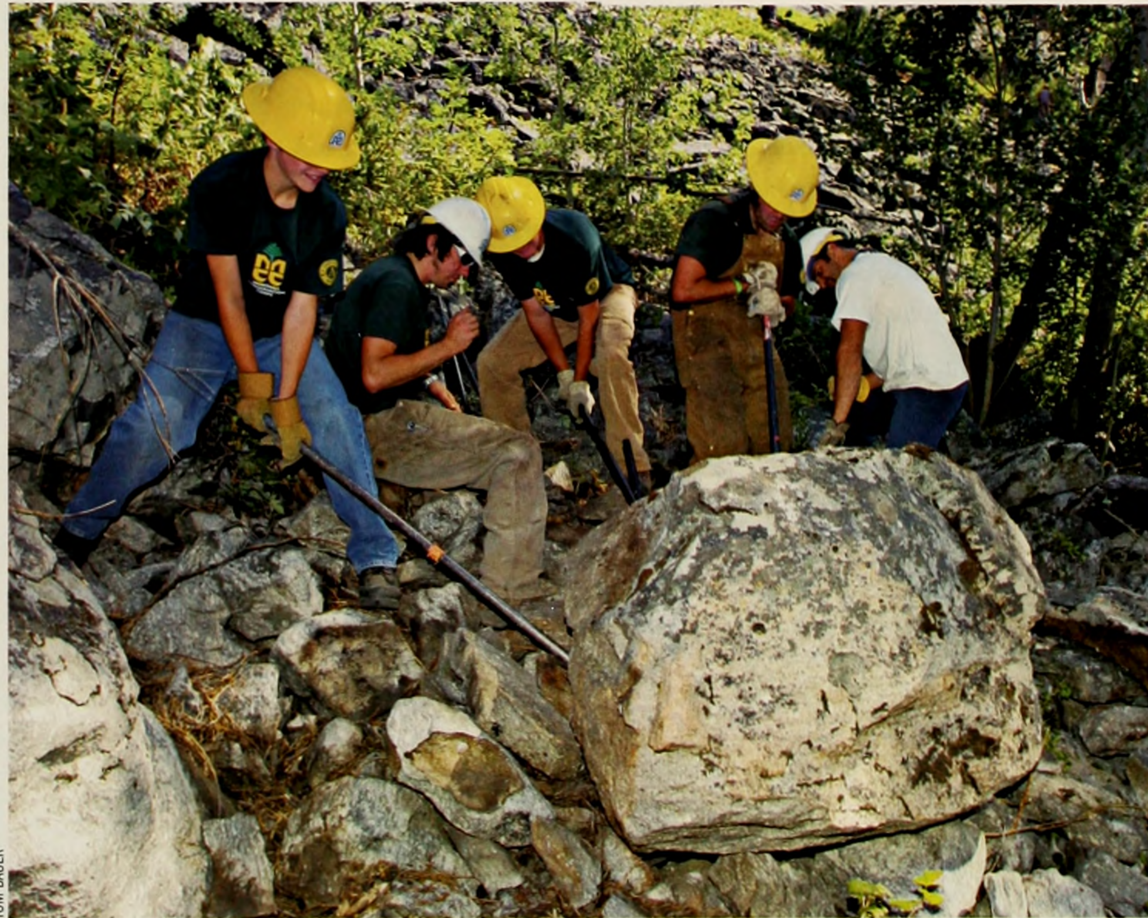
ROCK ON Dynamite dislodges the biggest boulders blocking trails, but MCC crews use their backs and spud bars to move the rest.
