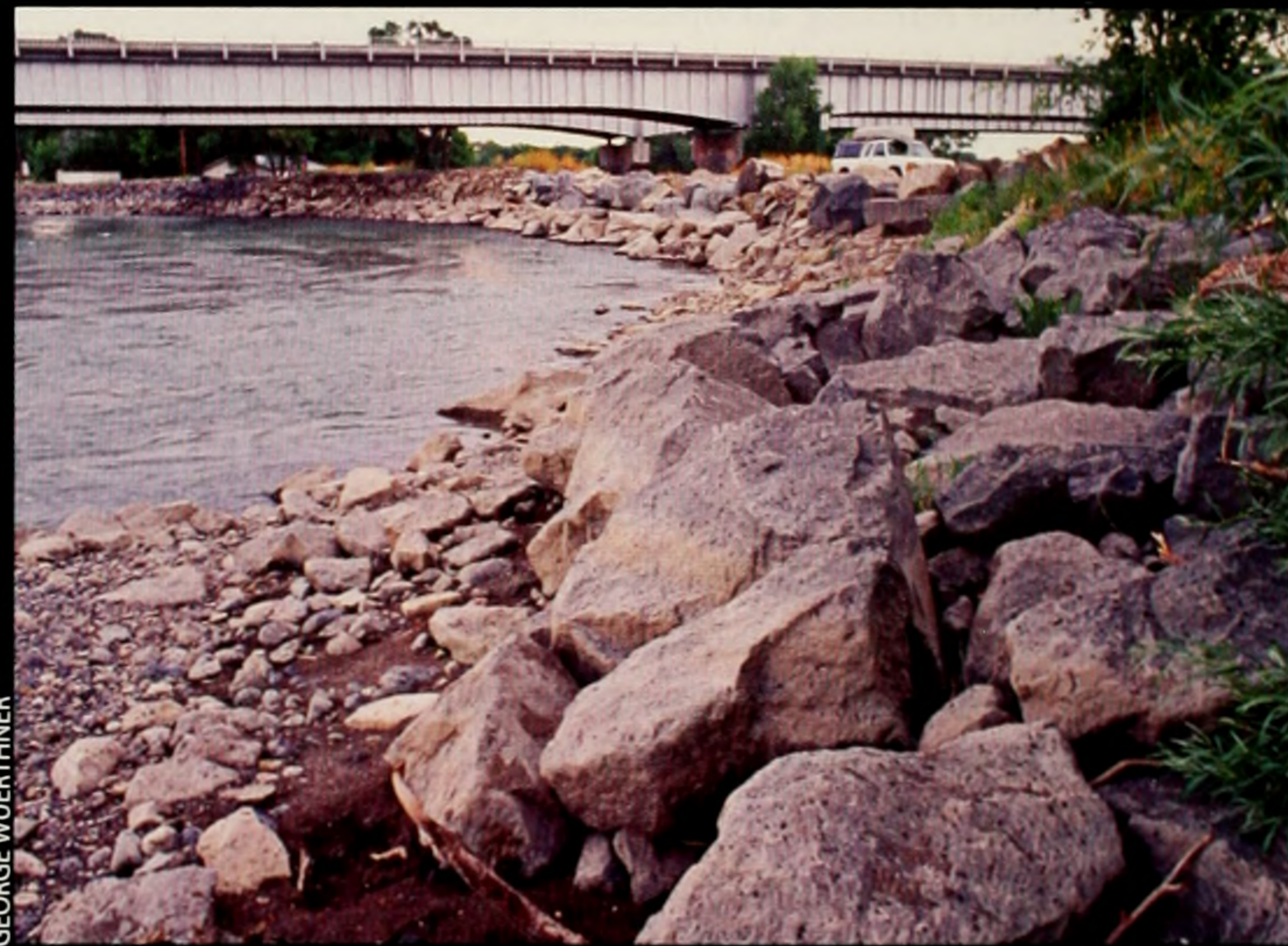
BETWEEN A ROCK AND A HARD PLACE Floodwaters must eventually spill out somewhere. By building dikes and armor-ing banks with riprap, communities and landowners squeeze the river and move flood energy downstream, where it creates even worse flooding for people there.
