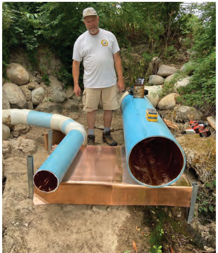
Copper covered strut channel and new copper lined and extended effluent plumbing 2022.
