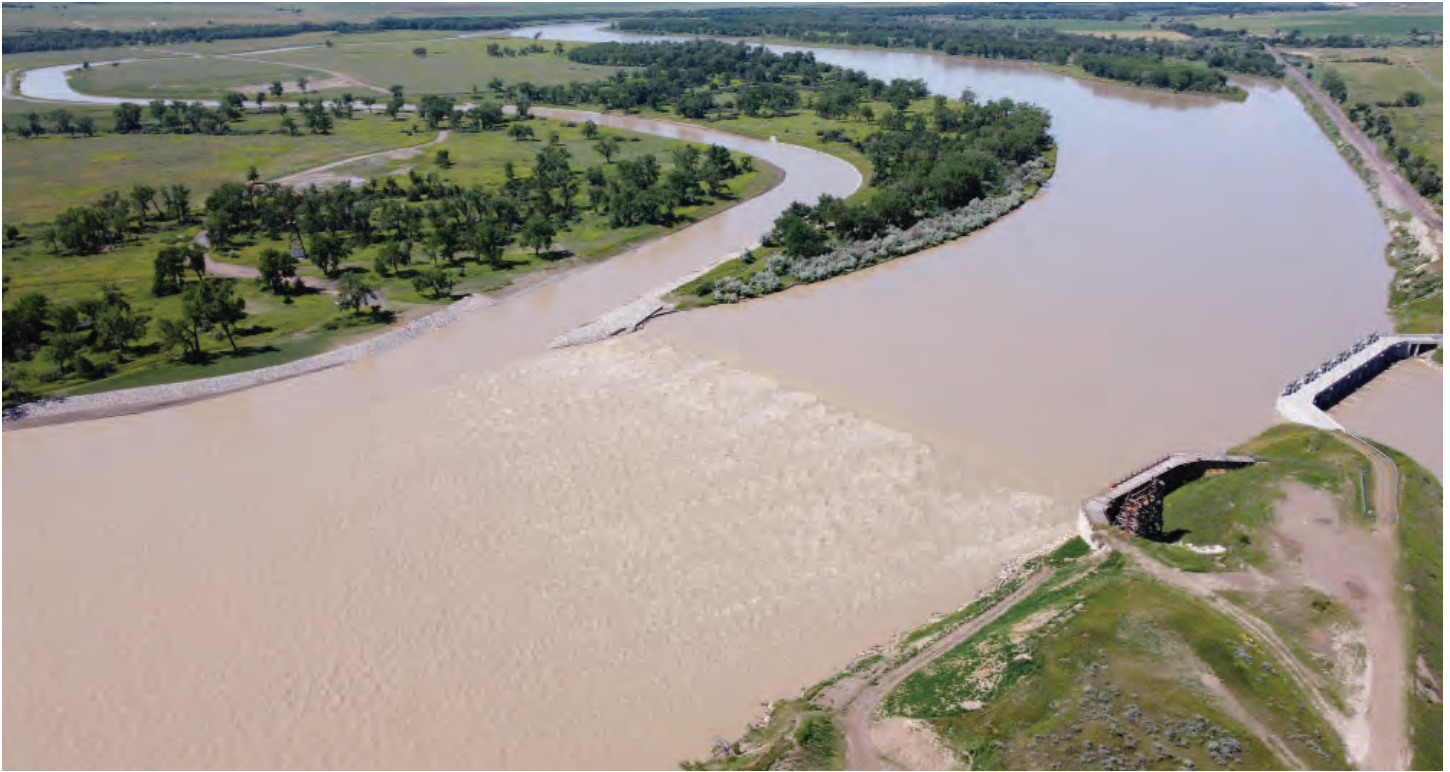
Intake Diversion Dam and Bypass Channel, provided by U.S. Bureau of Reclamation.
