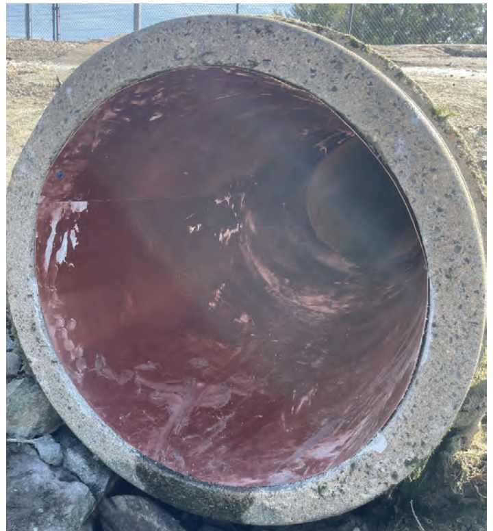
Newly installed copper lining in an outflow pipe.
