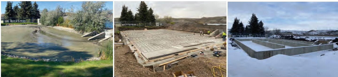
Settling pond before, during and after construction.
