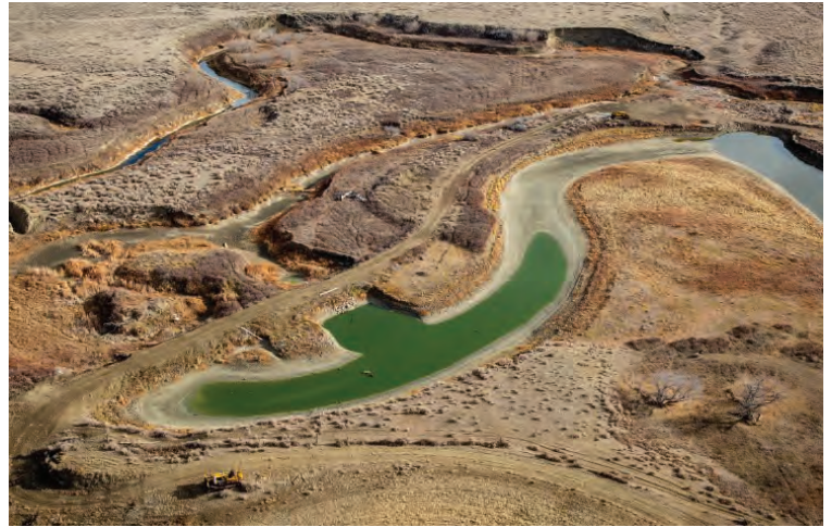
Example of an in-channel dam - Larb Creek, Valley County.
