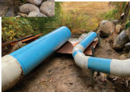
Copper covered strut channel and new copper lined and extended effluent plumbing 2022.
