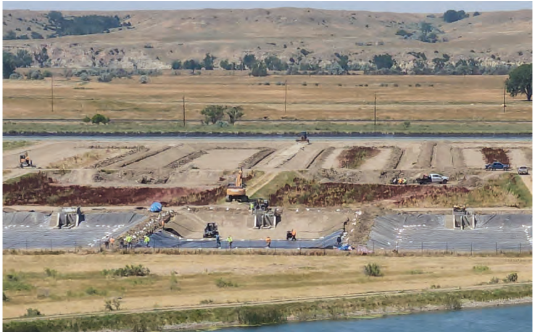
Pond liners being installed.
