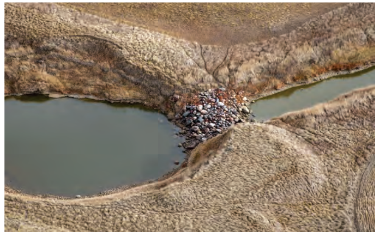
Example of a hardened crossing – Larb Creek, Valley County.
