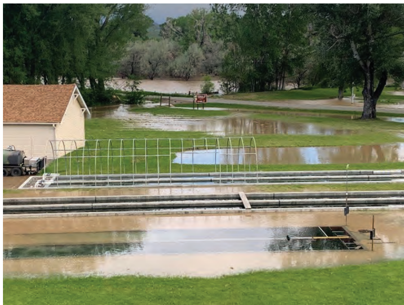
Early morning of the flood inundating only two raceways.
