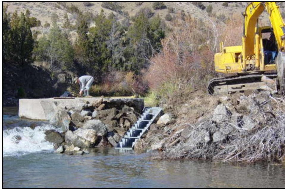
Photo Illustration 6. (Upper photo) Work crew preparing bundles of salvaged Christmas trees for placement in strategic locations in Canyon Ferry Reservoir. These tree bundles provide for spawning and rearing habitat for yellow perch, a very popular fishery in the reservoir. (Lower photo) Installation of a Denil style fish ladder located on the Boulder River east of the town of Whitehall. This ladder will provide for migratory passage over an existing irrigation diversion structure by spawning brown trout and possibly rainbow trout.
