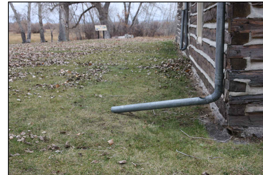
CHIEF'S HOUSE, EARTH SLOPING DOWN TOWARDS NORTH SIDE OF BUILDING
