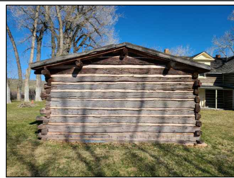
STORE EXTERIOR, SOUTH ELEVATION
